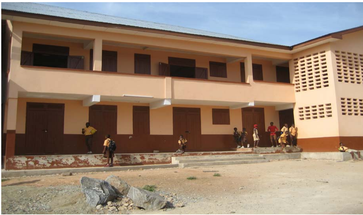
New Nima 1 School building opened in September 2010 under the auspices of the Ministry of Education financed by the GET Fund
